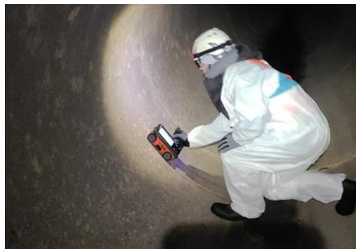
A SewerVUE technician performs PPR scanning.
